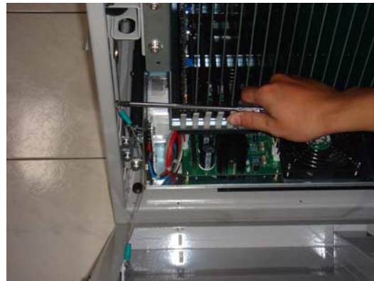
Figure 4 Unfasten supporting cables
